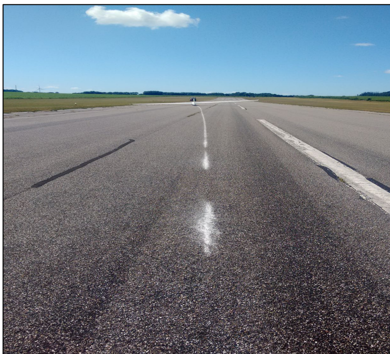
Photo no. 3: Scrape marks on the asphalt surface of runway 29.
