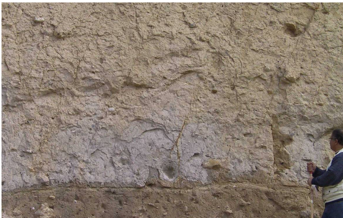
Figure 90. Sub-vertical fractures in clayey tills.
