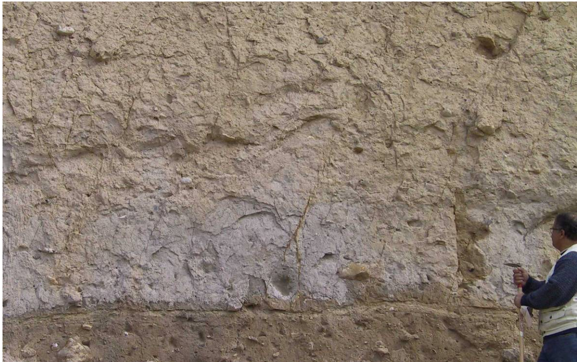
Figure 40. Section in clayey till with sub-vertical fractures (photo K.E.S.Klint).
