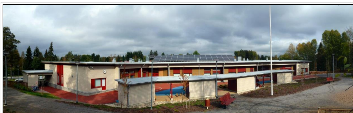
Figure 1: Luhtaa Day Care Centre in Tampere represents energy efficient modern construction.
