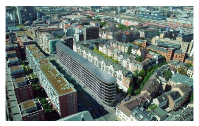
Figure 2: The Solar Active House in the city centre of Frankfurt features a heat pump coupled to the sewage water and PV modules on the roof and the façade (source: HHS Architekten).
