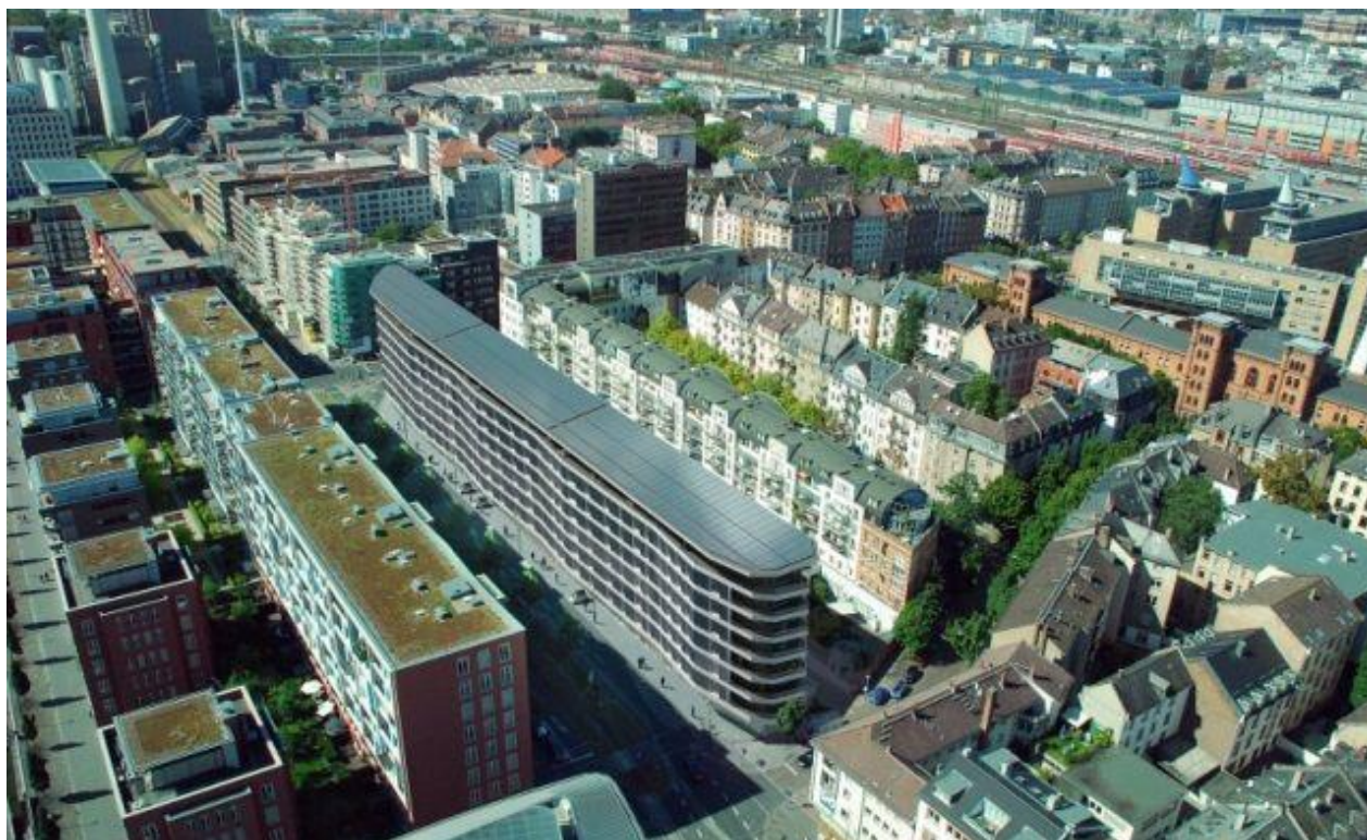
Figure 2: The Solar Active House in the city centre of Frankfurt features a heat pump coupled to the sewage water and PV modules on the roof and the façade (source: HHS Architekten).
